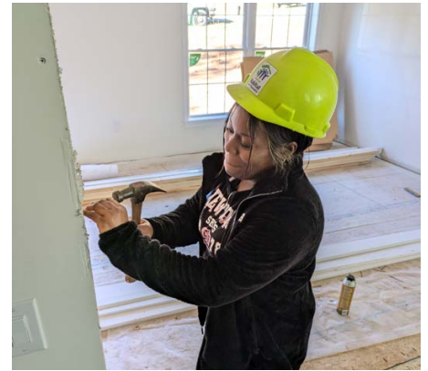
Shana on build site
